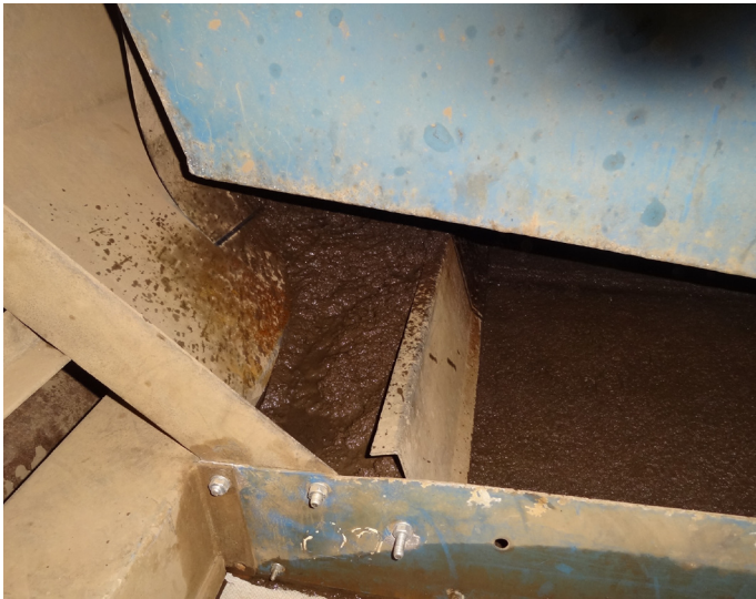
Sludge with high content of water/polymer filled in the belt filter.
