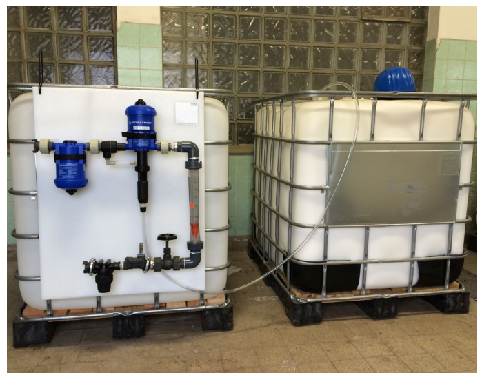
Pressed out water is running back in water recycling reservoir.
